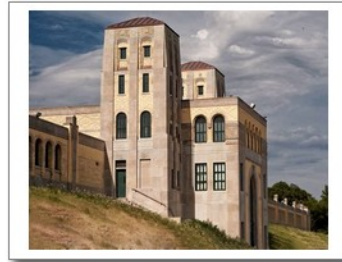
1035 Harris Water Treatment Plant
